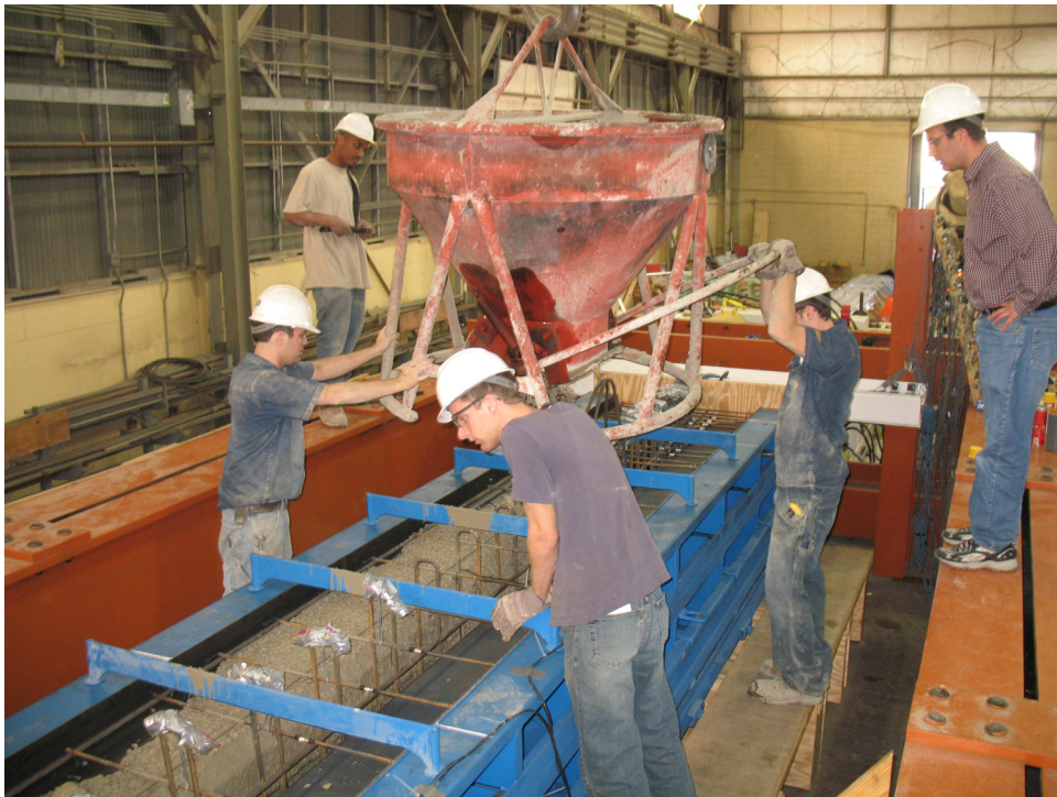
Figure 3- 13: Casting Operation for Tx Girder
