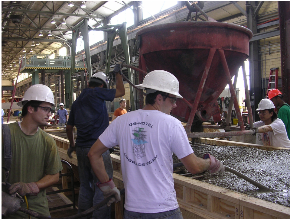
Figure 3- 19: Casting of composite concrete deck.
