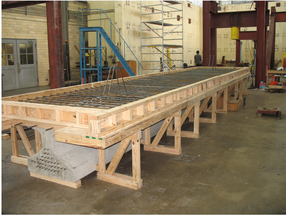
Figure 3- 18: Tx28 girder before casting of deck.
