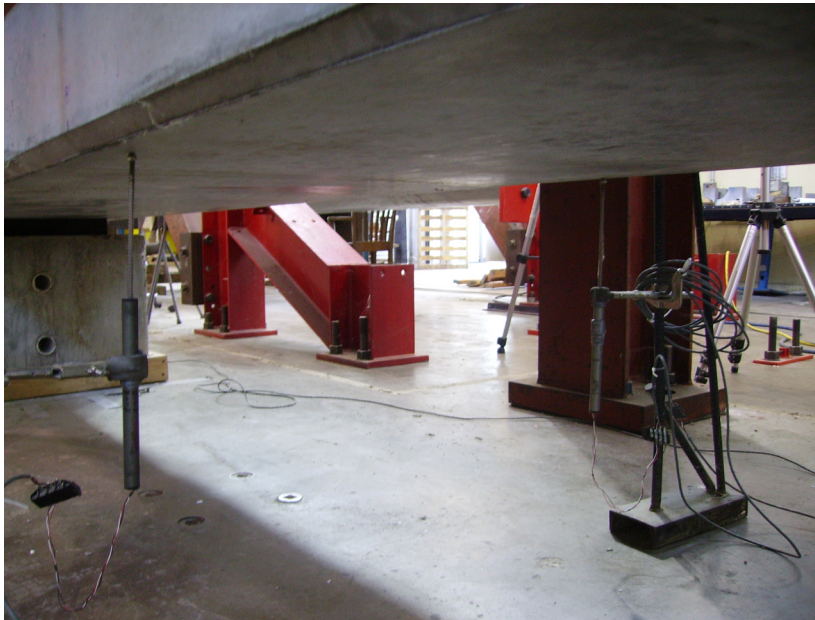
Figure 3- 10: 6" inch Linear Potentiometers at each side of the bottom flange under the load point.
